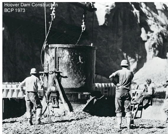
Pouring of concrete during the construction of Hoover Dam http://www.savelakemead.com/jpgs/hib/hib003fsConcretePour.jpg
